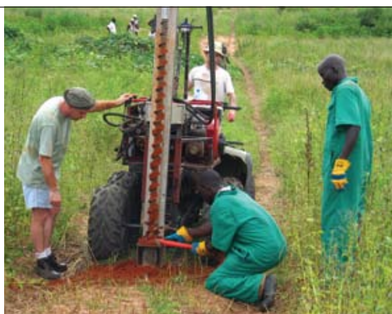
A 2-D seismic program was shot in Exploration Area 5 in Uganda to assess hydrocarbon potential.
