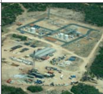
RIGHT AND OPPOSITE PAGE The new SS-10 well was drilled adjacent to the Songo Songo gas processing plant.
