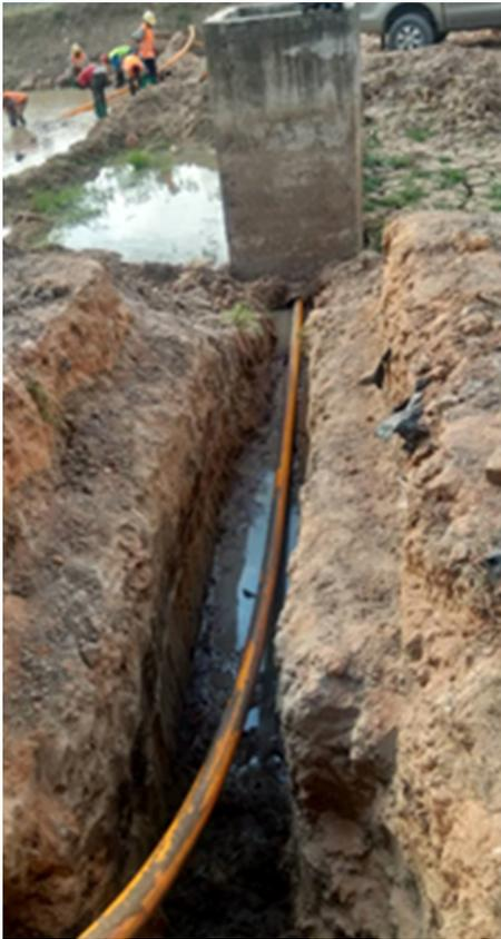
Running HDPE through inspection chamber.
