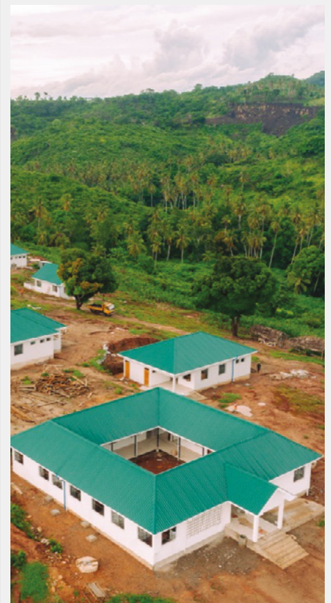
Construction in progress at Chumo Health Center
