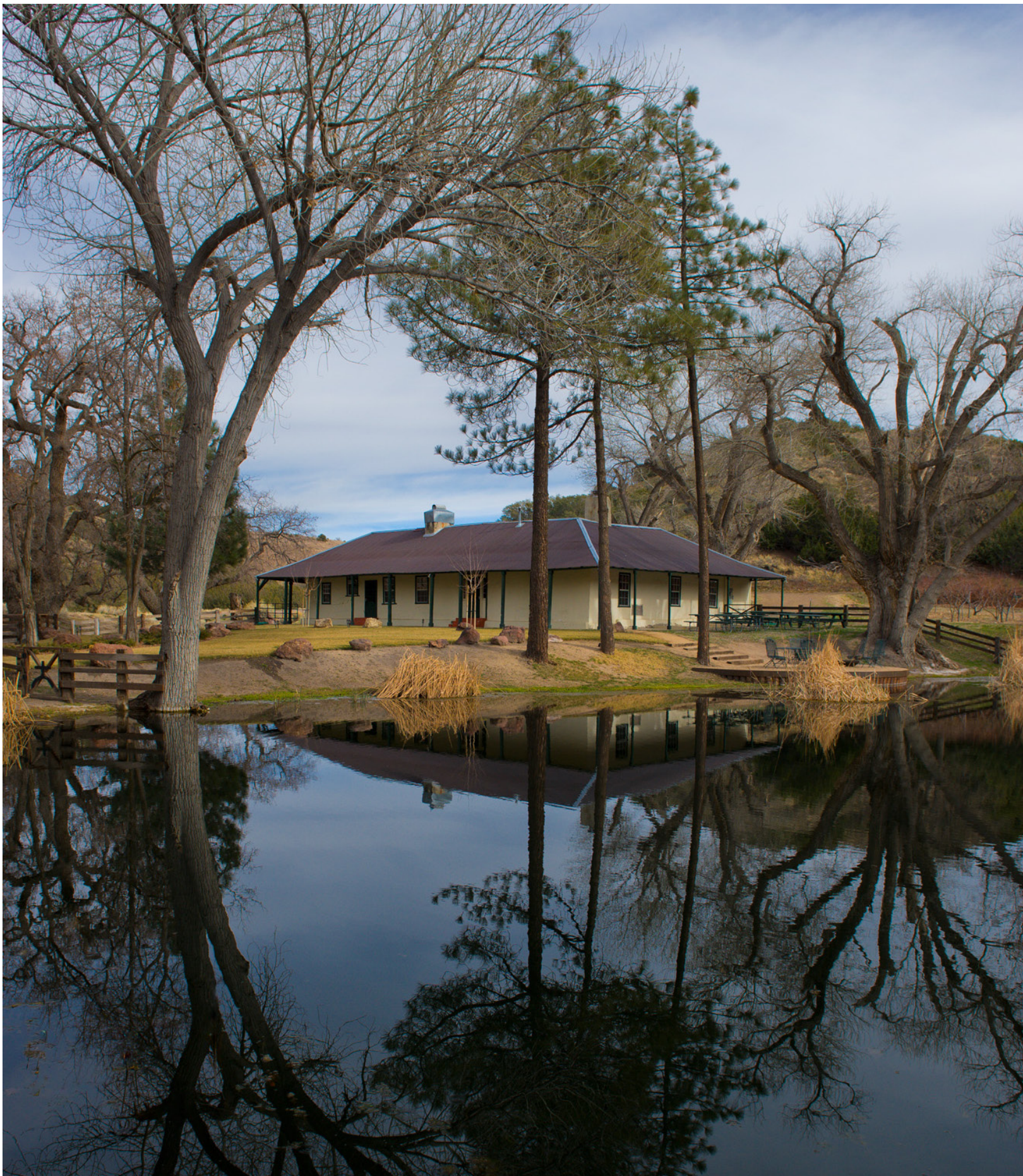
THE BEALE ADOBE, named for the founder of Tejon Ranch, Gen. Edward F. Beale, is located in the southern portion of the Ranch in the original La Liebre land grant. Built in the 1860s, it is the oldest building in the Antelope Valley.
