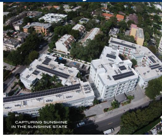
Hersha recently installed 336 Solar PV panels on the roof of its Residence Inn by Marriott Coconut Grove property in Florida. The system captures renewable energy from the sun and will generate over 150,000 kWh of electricity each year for use by the hotel.
