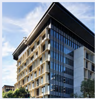
22 Cordelia Street, South Brisbane, QLD 100kW Solar PV System
