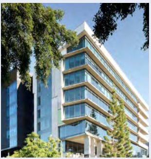
52 Merivale Street, South Brisbane, QLD 93kW Solar PV System
