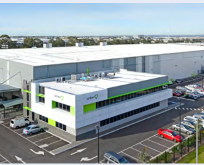
120-132 Atlantic Drive, Keysborough, Victoria 330kW Solar PV System
