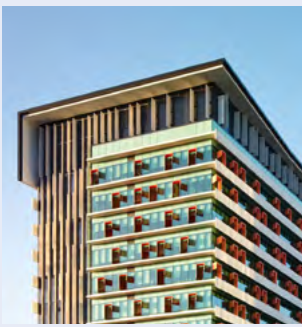
15 Green Square Close, Fortitude Valley, QLD 66kW Solar PV System
