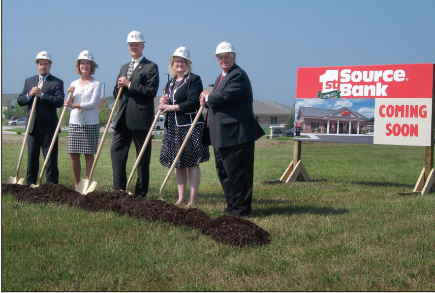
Luke Squires, Jan Wilhelm, Larry Mayers, Deb Moser and Jim Seitz at the ground breaking of the Illinois Road Banking Center in Fort Wayne.
