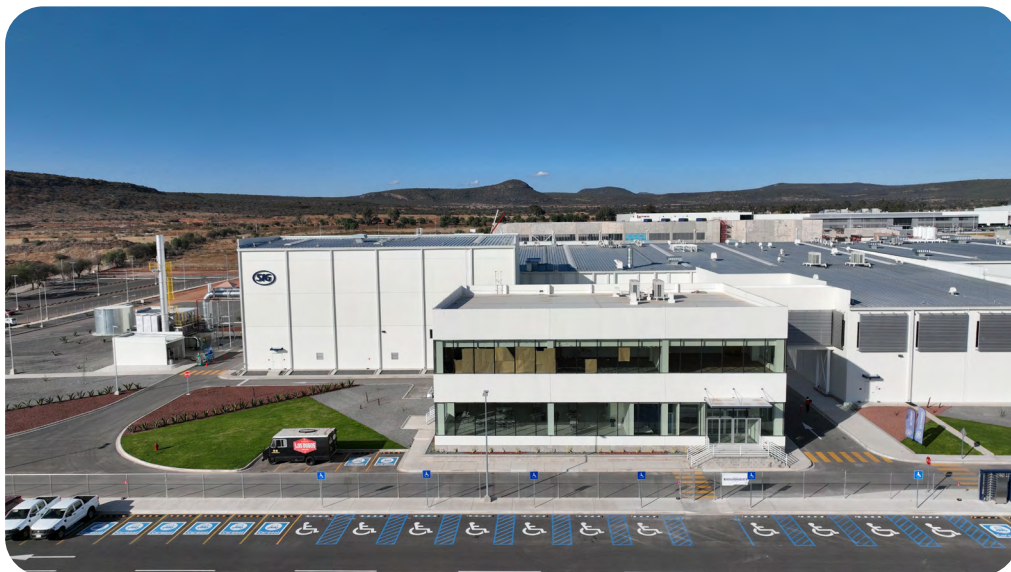
Our first aseptic carton packaging plant in Mexico.
