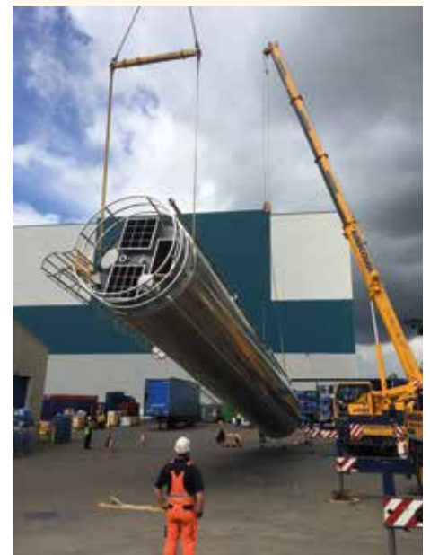
The sugar dissolver silo is installed.
