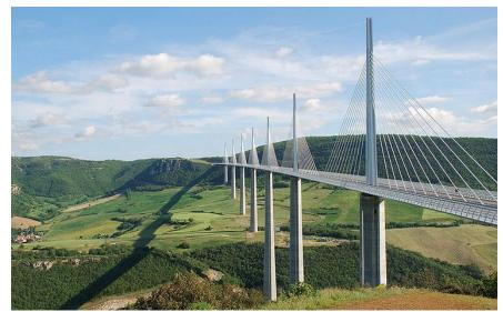
The addition of 0.0025% of Niobium to the steel in the Millau Viaduct reduced the weight of the steel and concrete by 60% in the overall project (Source: CBMM)
