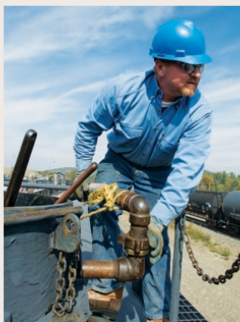
Inergy’s Bath LPG storage facility, located on 125 acres near Bath, New York, has high-performance rail and truck loading facilities.
