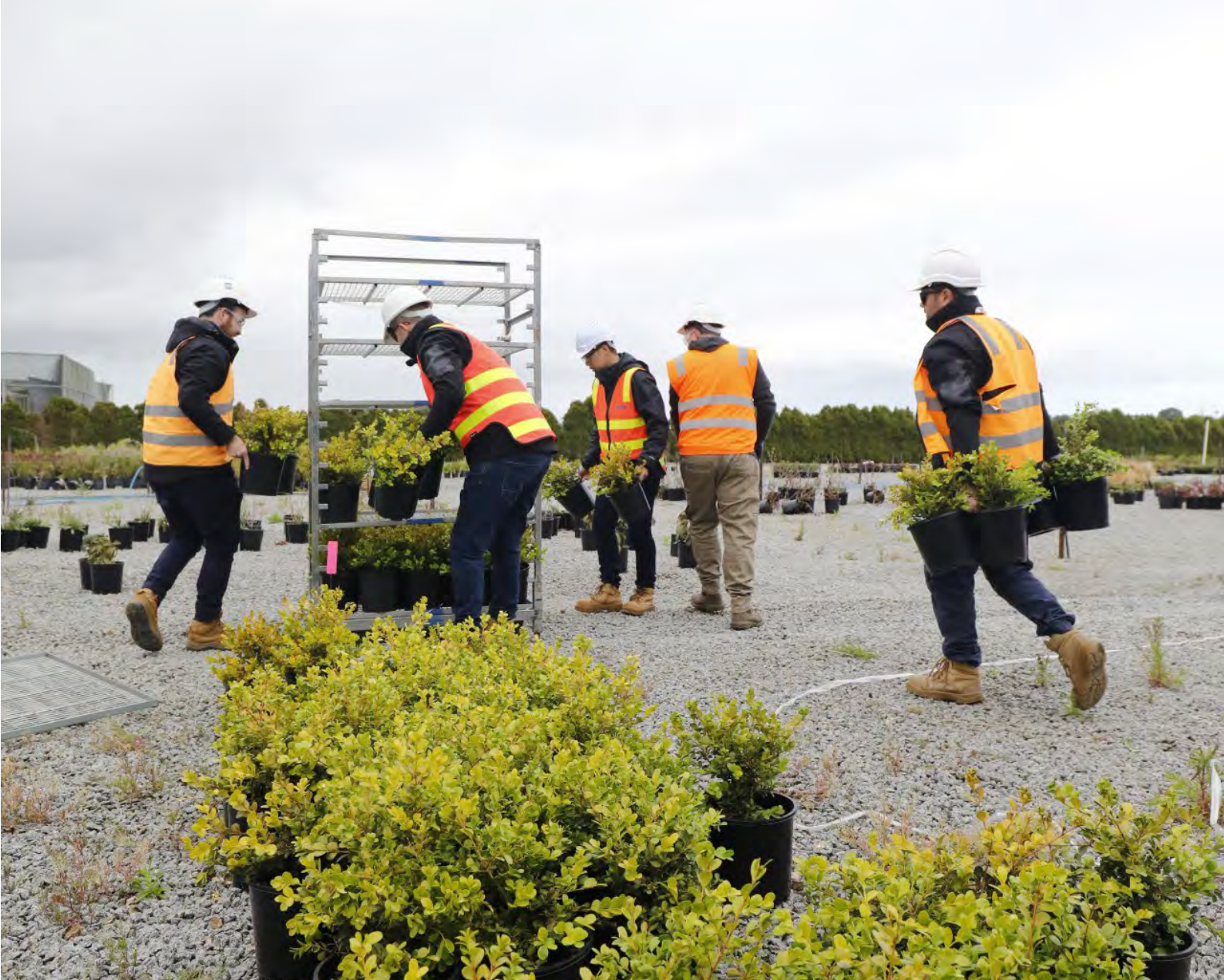
Mordialloc Freeway Project South-East Melbourne, Victoria
