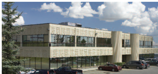
Calgary, Franklin Atrium
