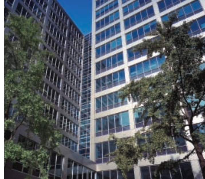
30 ADELAIDE STREET EAST, TORONTO Dundee was responsible for the innovative redevelopment of an obsolete and vacant property, creating a new downtown office complex with suburban campus amenities at an affordable price.
