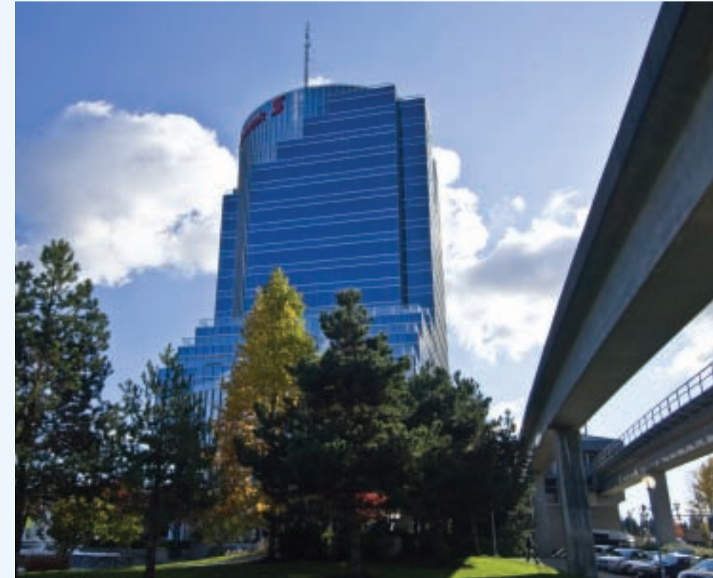
Station Tower Surrey, British Columbia
