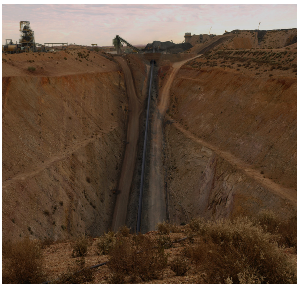
NCO - Box Cut
