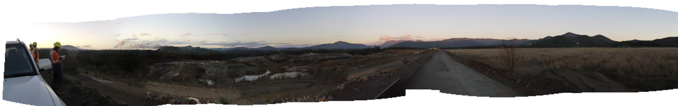
Tailings Storage Facility
