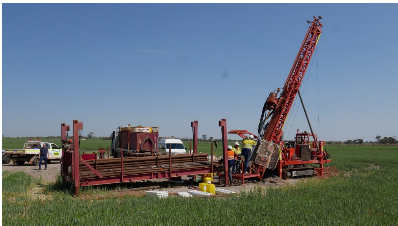
Figure 19 – Diamond drill rig at the Wyatt’s prospect.
