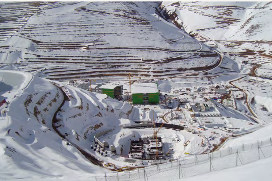
▲ Caserones Project. Chile
