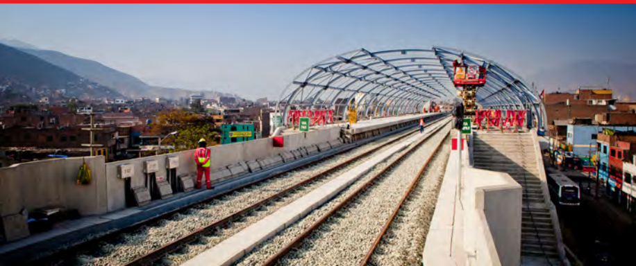
▲ Construction of tranche 2 of Metro of Lima
