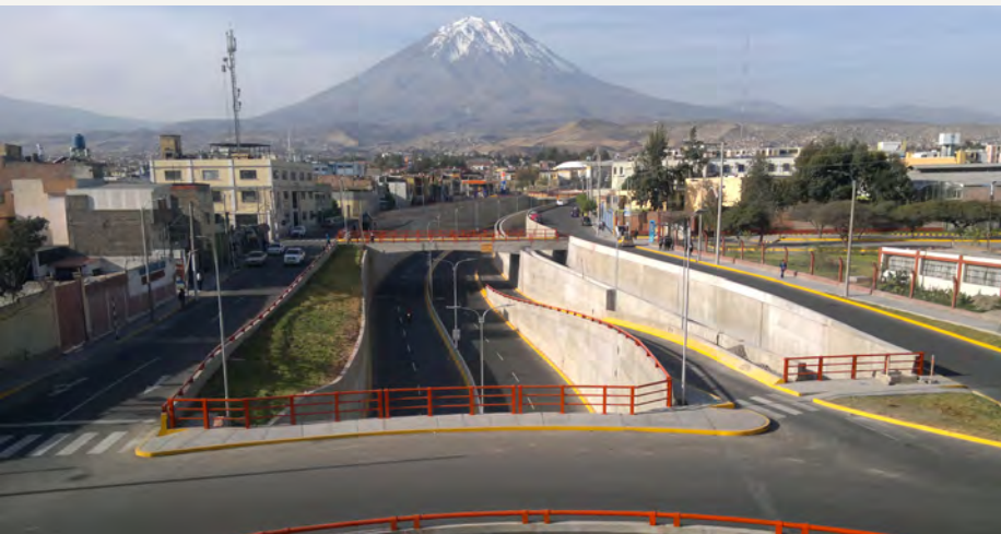
▲ Palomar road Exchange in Arequipa
