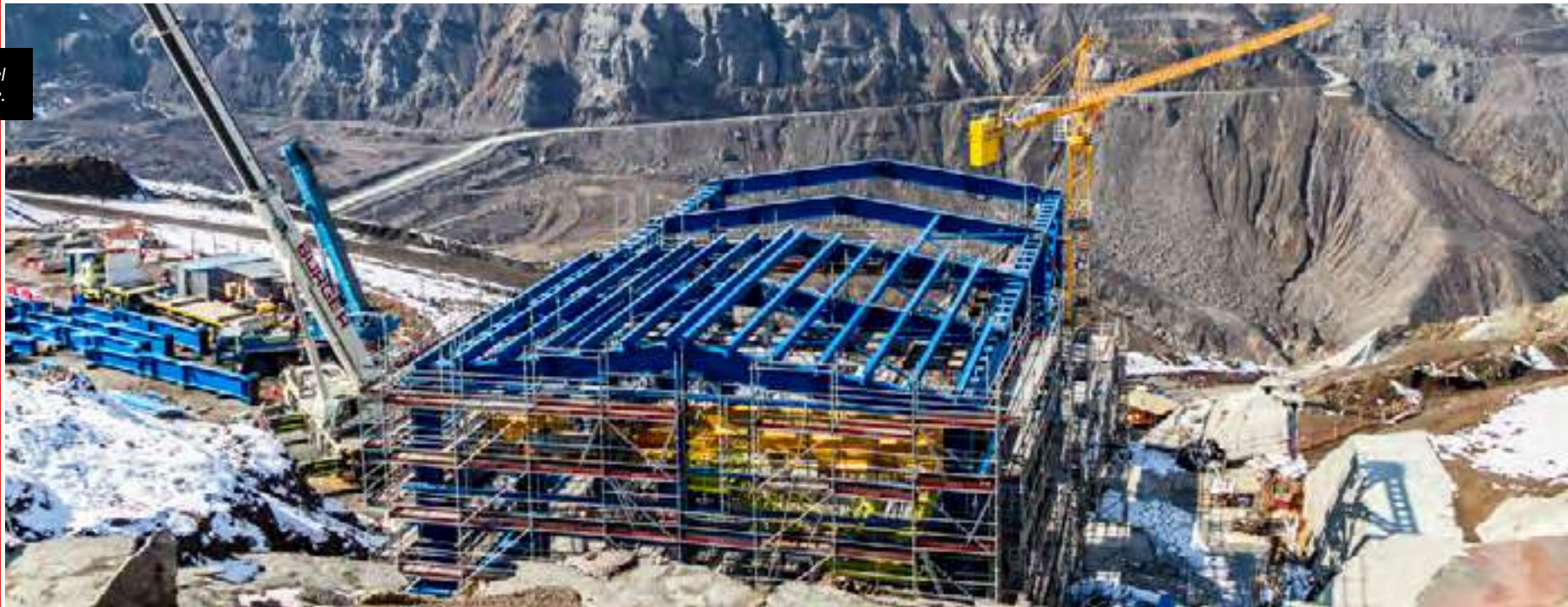
New Mine Level Project, Rancagua, Chile.
