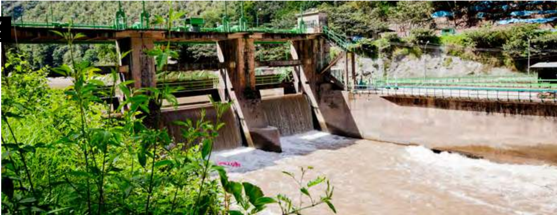
Machu Picchu Hydroelectric Station, Cusco, Peru.
