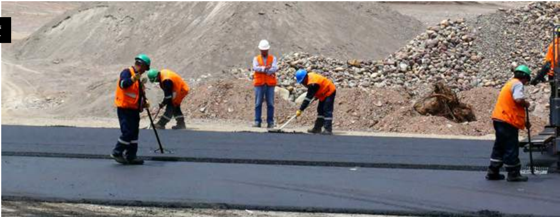
Maintenance of Urcos Beltway, Cusco - Peru.
