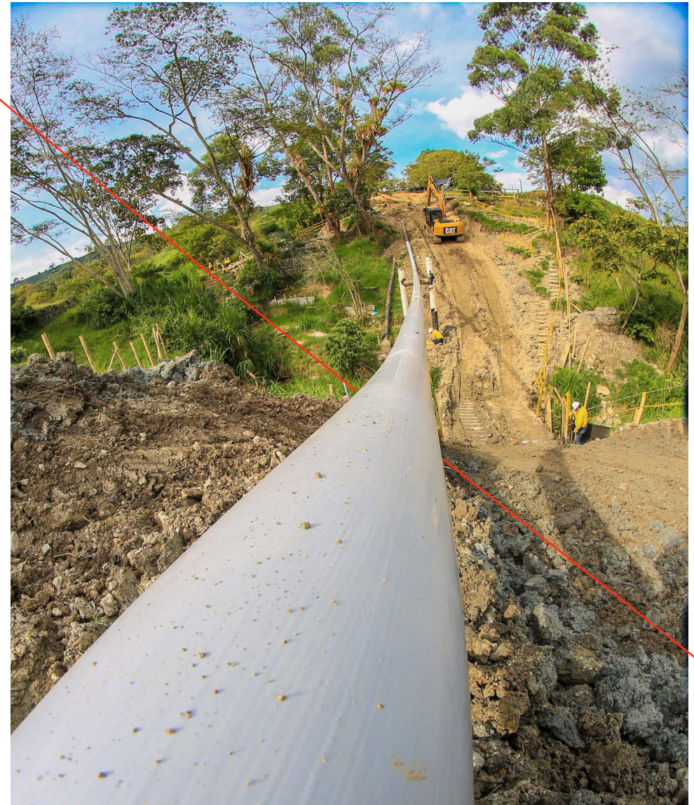
» Oil Pipeline Maintenance Colombia
