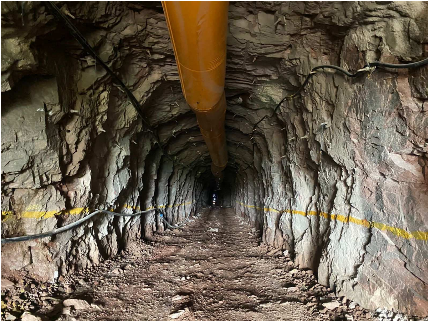
Figure 8- Initial ramp development at Coringa
