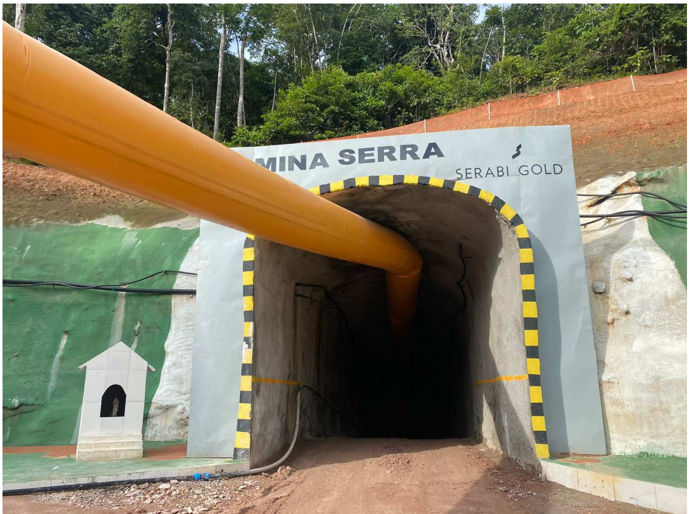
Figure 7- The Coringa mine portal
