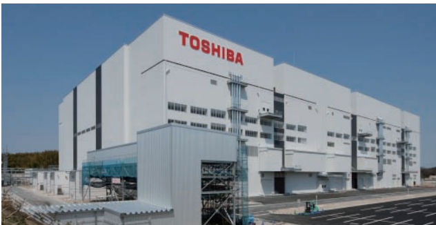
Yokkaichi Operations has completed construction of its Fab No.5 wafer production facility. Production started in July 2011.
