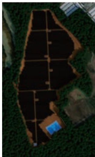
Ikeda Solar Power Plant
