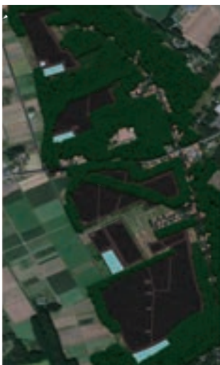
Yatsubo Solar Power Plant
