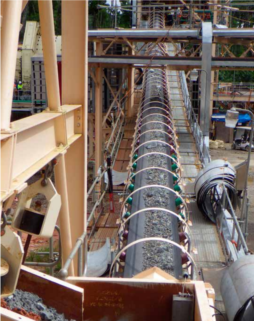
Photo 1: Crushed ore being loaded into Sag Mill
