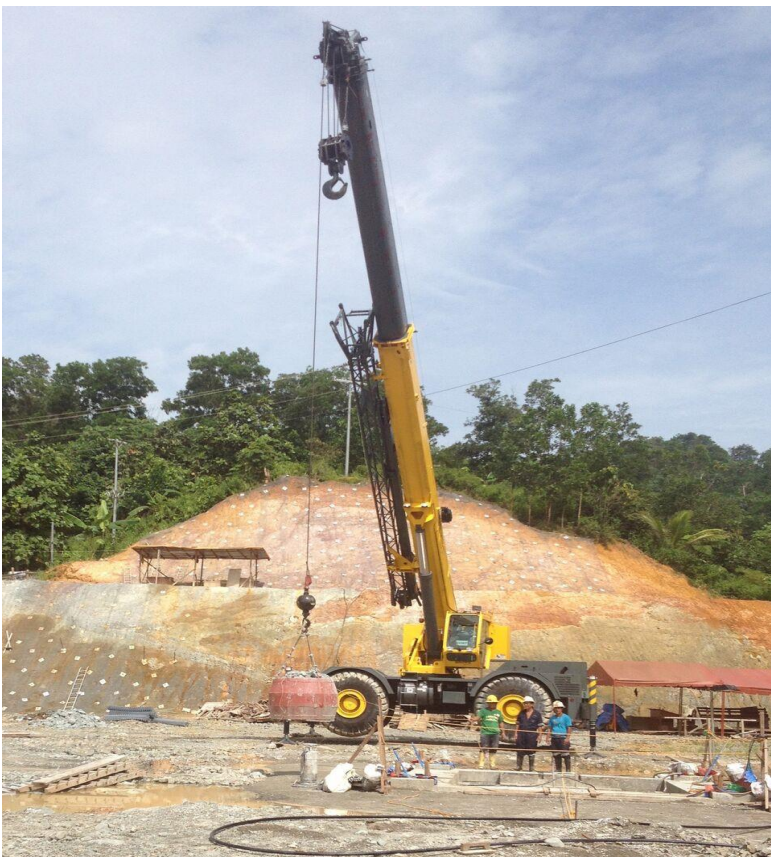
Photo of Service Shaft collar currently being excavated.
