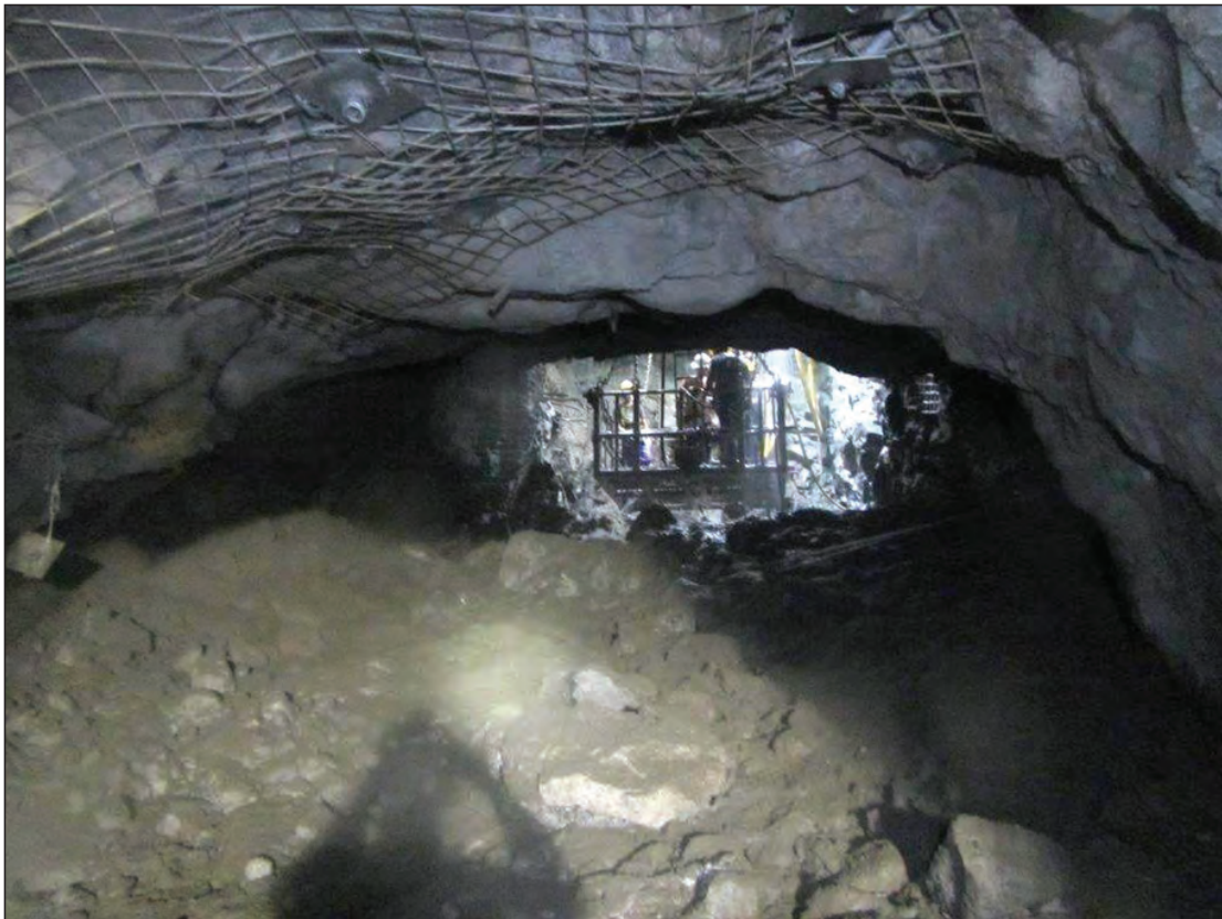
Picture 4: Shaft break through onto 5 Level
