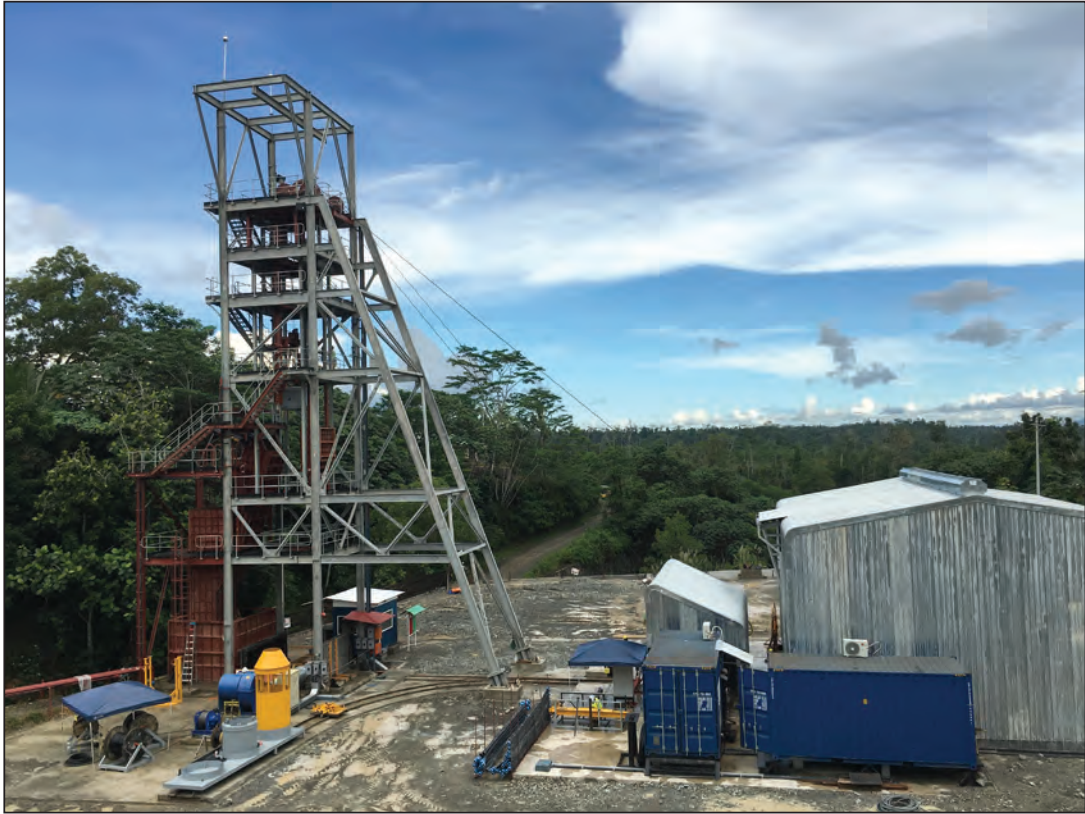
Picture 3:: E15 Head Frame and winder houses
