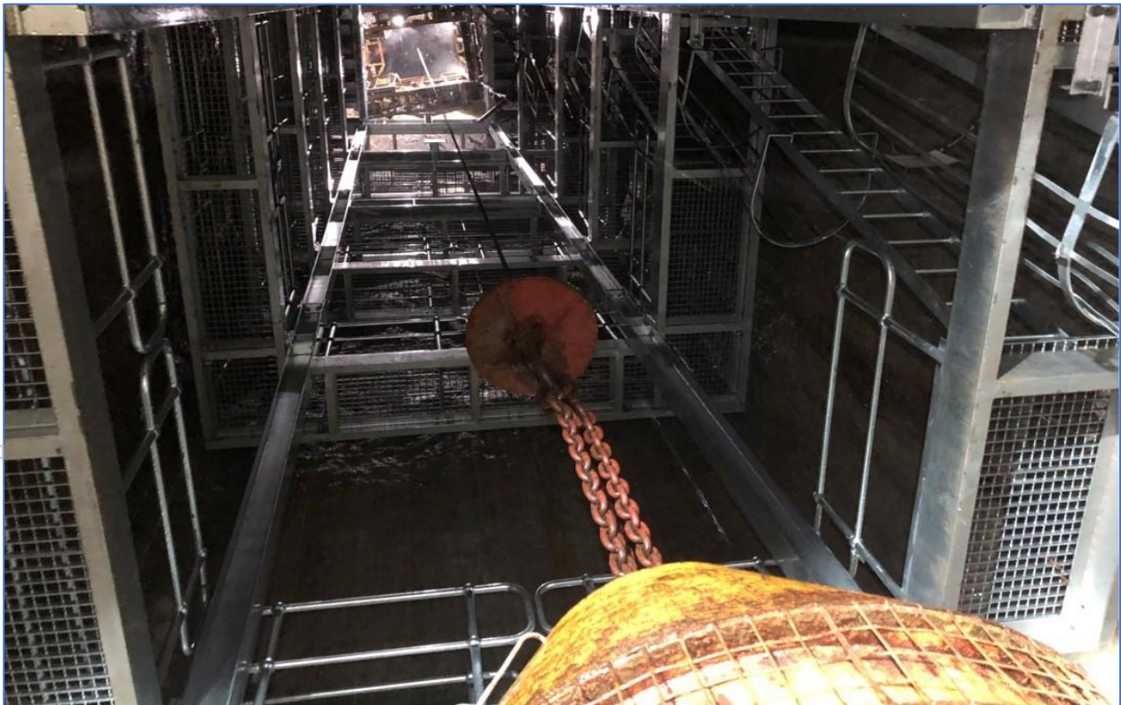
Picture 3: Current progress of E15 Service Shaft installation.
