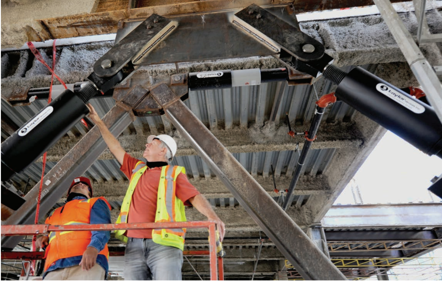
Pete Silva (left) of Olson Steel and Buzz Harwood (right), Taylor Devices' representative, inspect the damper installations inside the One Westside building.
