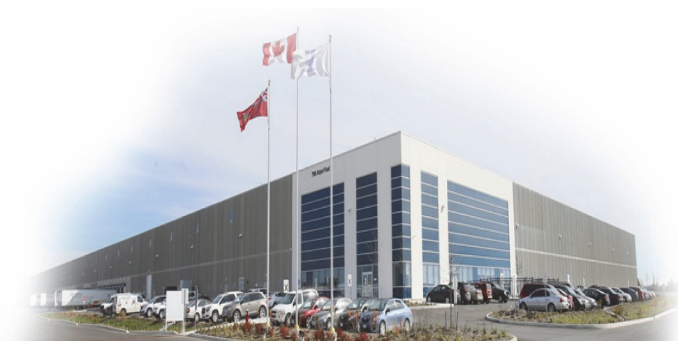
Airport Road, Brampton – Unilever Distribution Warehouse
