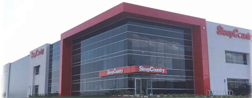
Airport Road, Brampton – Sleep Country
