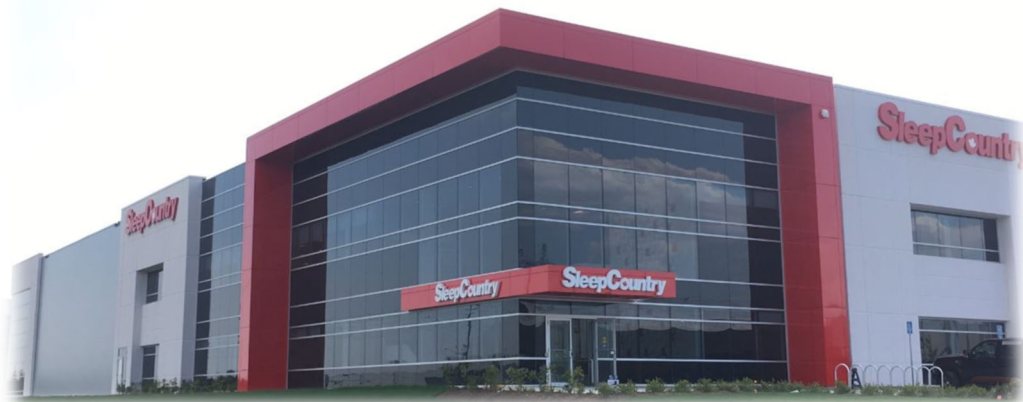
Airport Road, Brampton – Sleep Country
