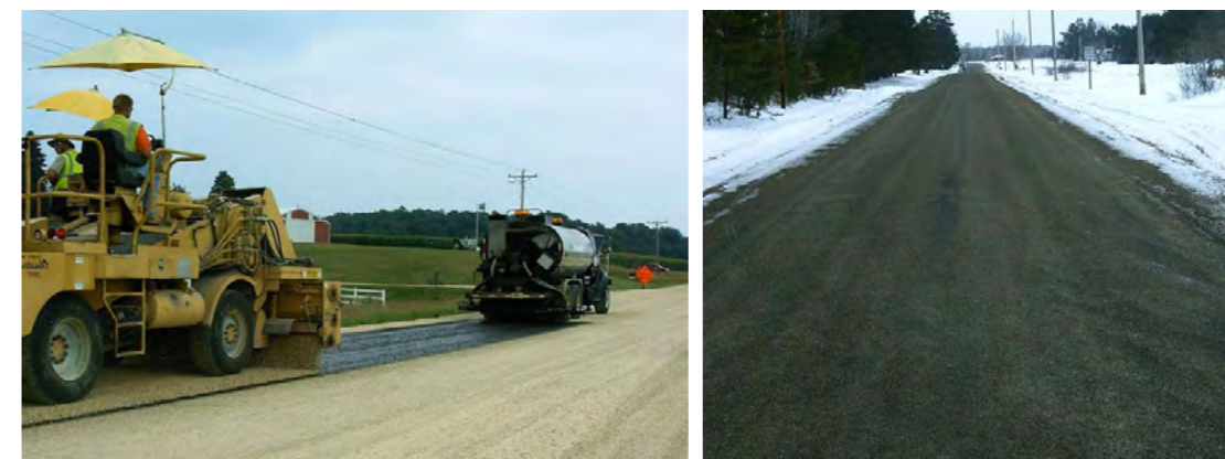
Above: Otta Seal Construction (2007) and finished road.
