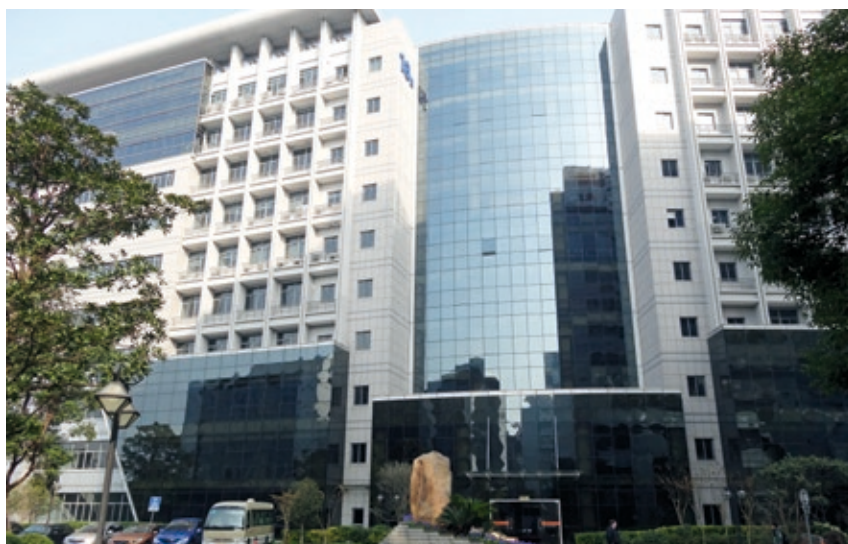
New 34,400 sq ft headquarters over two levels at the Shibe Hi-Tech Park in Shanghai's Zhabei district.
