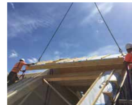
Fitting Smartroof panels at Goetre Uchaf, Bangor
