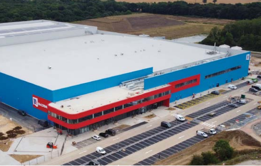
Completing our U.K. Flavor Solutions net-zero manufacturing facility, which will be operational in 2022.
