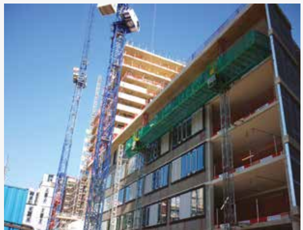
THE FILAMENTS, SW18 New business centre opening in Wandsworth.
