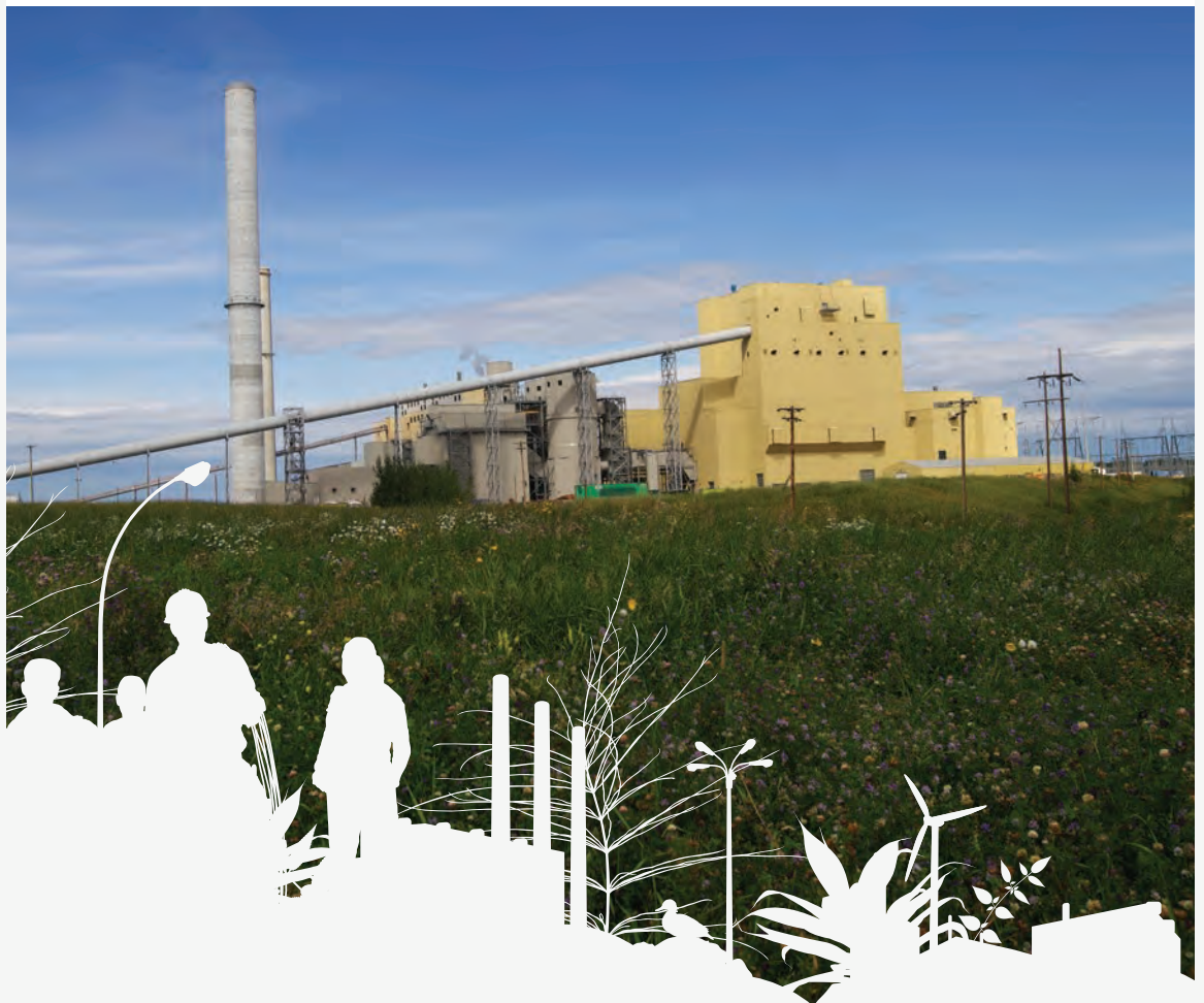
Keephills 3, located west of Edmonton, Alberta
