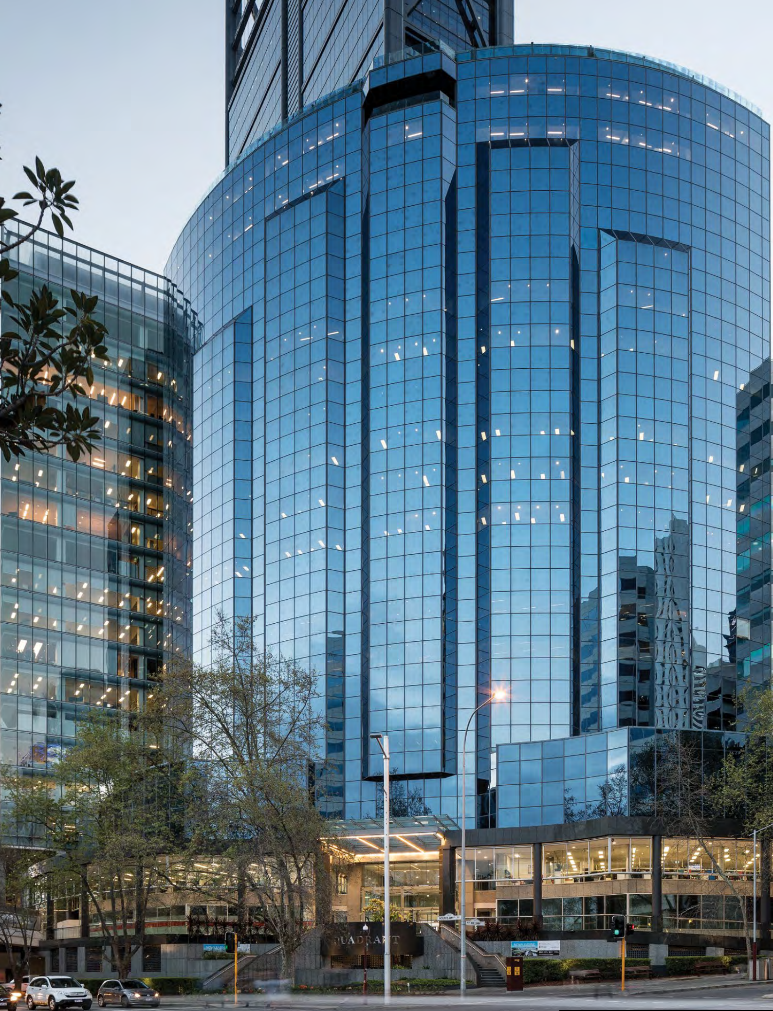
UNLISTED: 1 WILLIAM STREET, PERTH, WA
