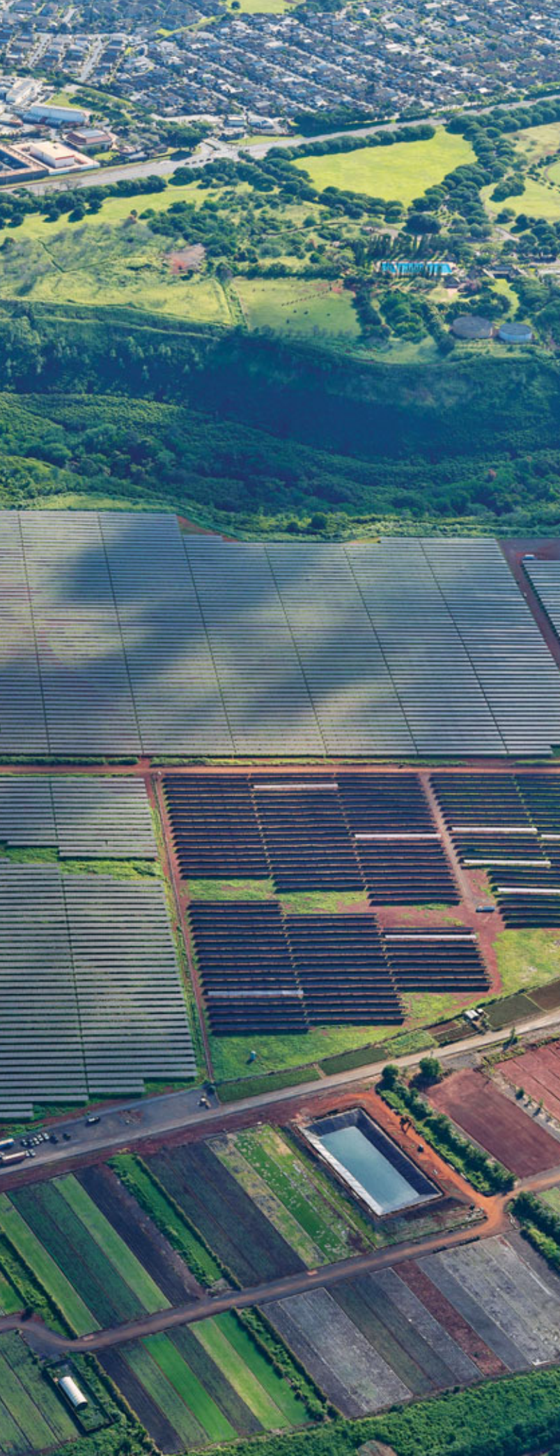
Left: Mililani I Solar, a 39-MW/156-MWh solar-plus-battery storage project, came online in July 2022. Photo courtesy of Clearway Energy and Moss Solar.
