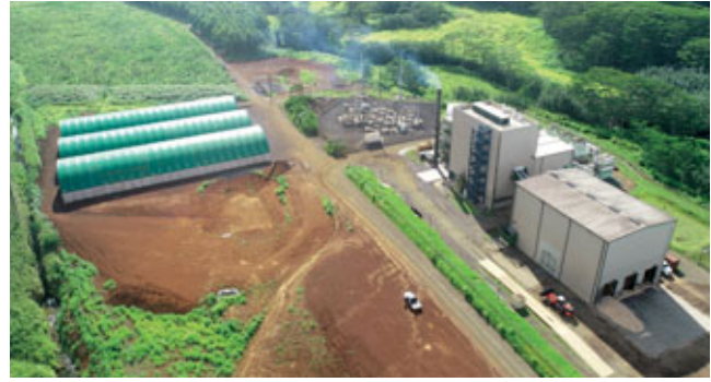
Pacific Current's newest addition is the Mahipapa biomass plant, which provides nearly 7 MW of firm renewable energy to Kaua'i residents. The plant is located in Kōloa, surrounded by the eucalyptus trees that power the facility.
