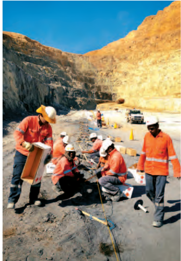
Sukari blasting team charging pre-split holes
