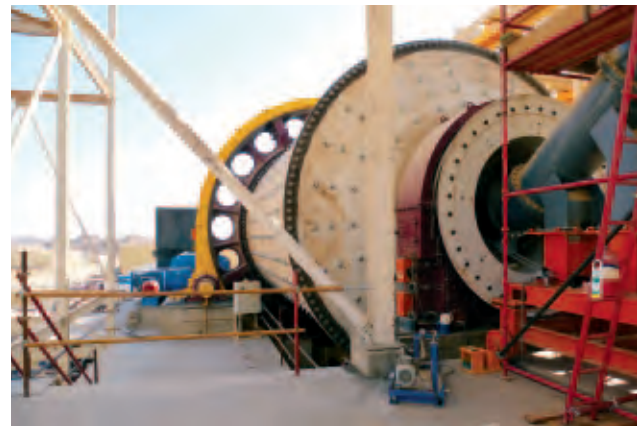
Stage 4 expansion plant with new SAG Mill in place
