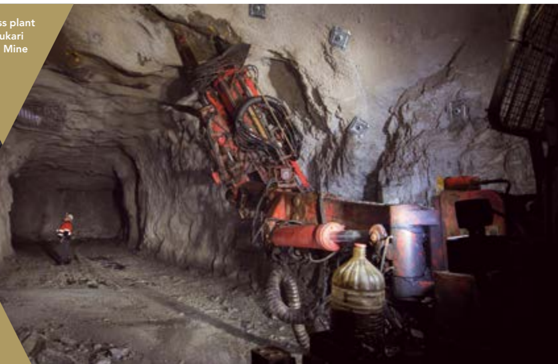
Underground development drive
