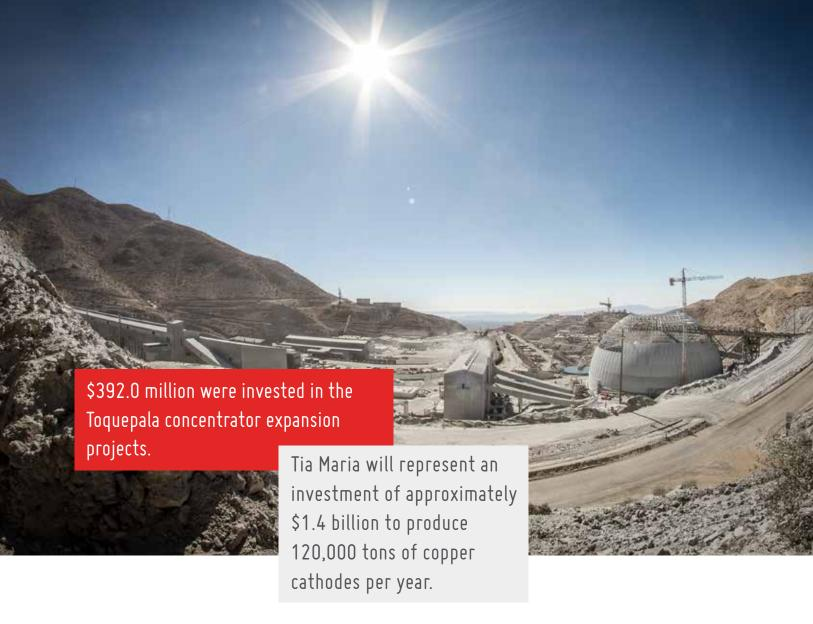
The new copper-molybdenum concentrator has an annual production capacity of 188,000 tons of copper and 2,600 tons of molybdenum. The project will additionally produce 2.3 million ounces of silver and 21,000 ounces of gold per year. The total capital budget of the project is \$1,383.6 million and as of December 31, 2015, the project had a 99% progress with an investment of \$1,162.0 million.
