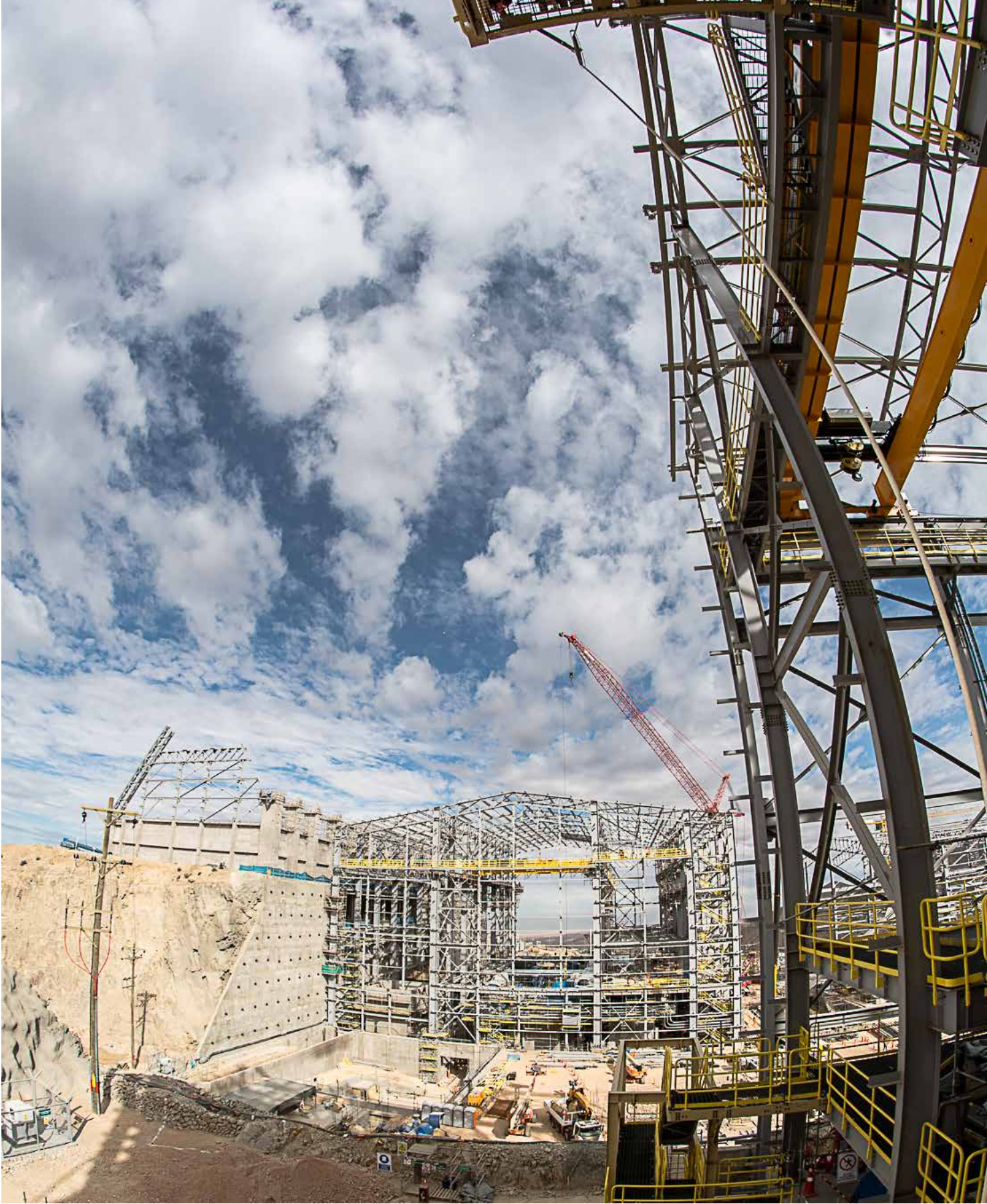
Progress in the Toquepala Concentrator Expansion, Tacna, Peru.
