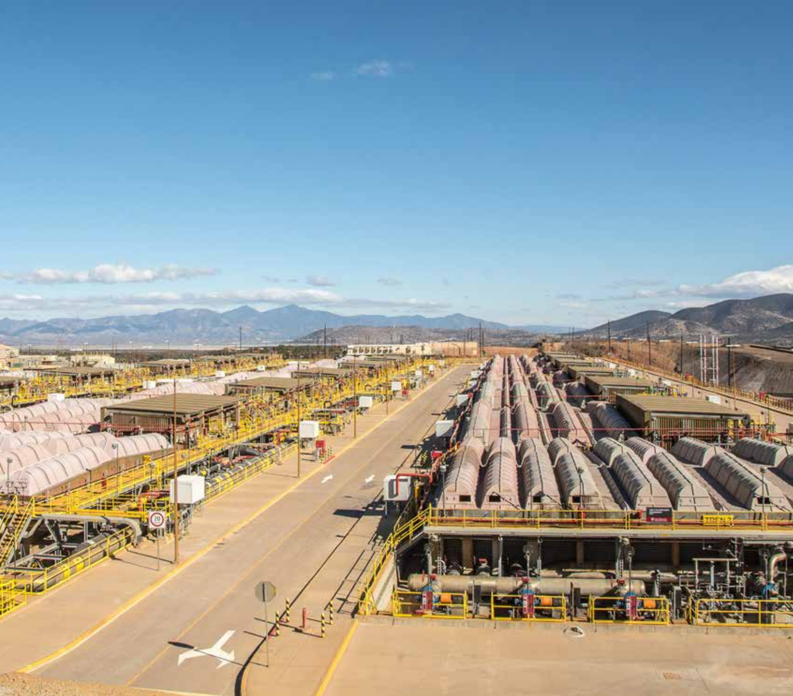
SX-EW III Plant, Sonora, Mexico //
