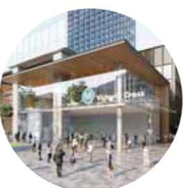
Victoria Cross over station development, Sydney
