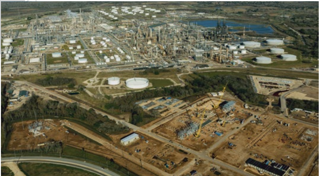
| Sweeny Fractionators II and III Construction OLD OCEAN, TX
