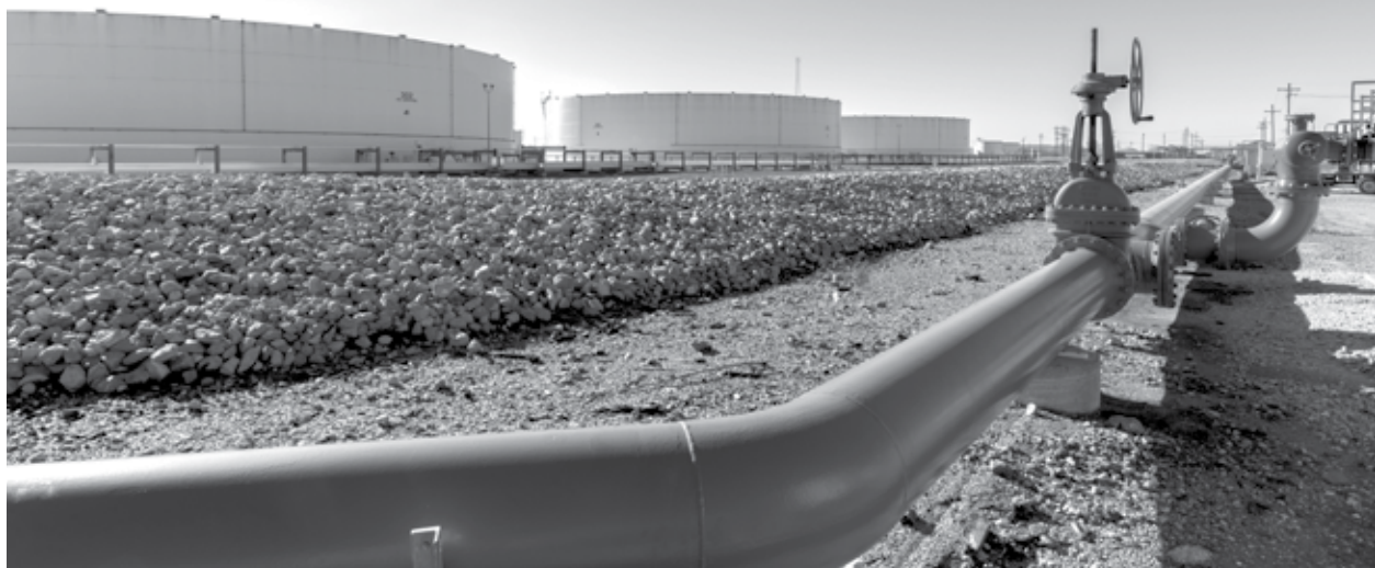
| Beaumont Terminal Methanol Storage Tanks NEDERLAND, TX
