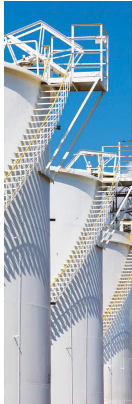
| Lake Charles Refinery Gasoline Storage Tanks WESTLAKE, LA
