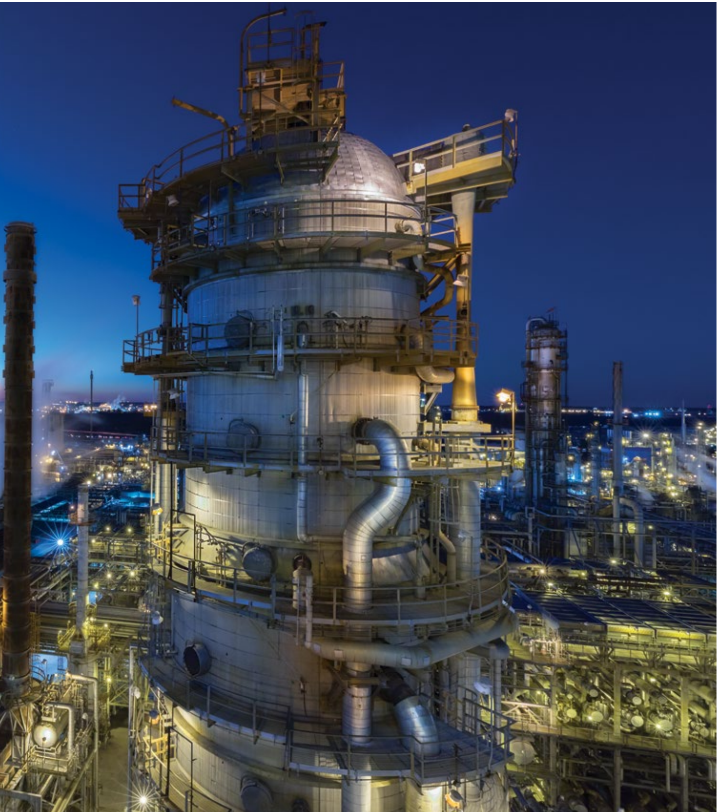
| Lake Charles Refinery Fuels Coker and Premium Coker Derricks, Excel Paralubes Joint Venture Vacuum Tower LAKE CHARLES, LA
