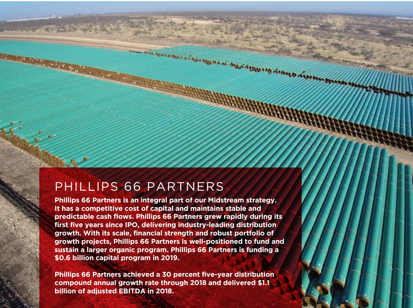
| Gray Oak Pipeline Construction Pipe Yard BIG LAKE, TX
