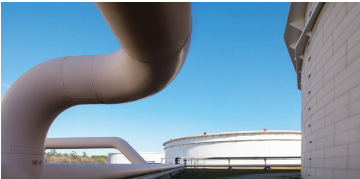
Clifton Ridge Marine Terminal SULPHUR, LA
