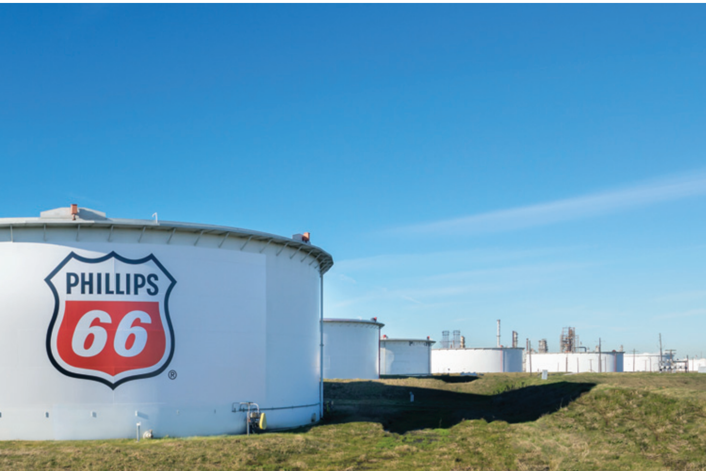
Lake Charles Refinery Storage Tanks WESTLAKE, LA
