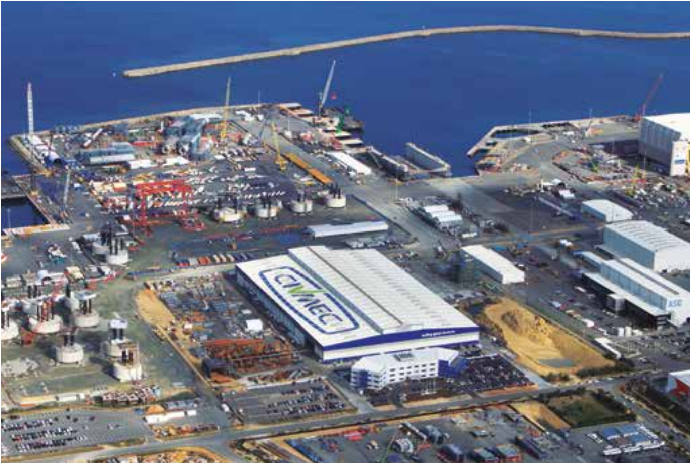
Civmec's new 6,500m 2 four storey 'state of the art' office in Henderson, Western Australia, is fully equipped to a high standard and can accommodate over 450 personnel. Facilities include: Training and induction centre, medical centre with a qualified nurse for onsite first aid and pre-employment medicals, boardroom and meeting rooms with video and conferencing facilities and fully serviced Client offices.
