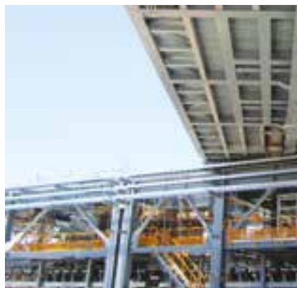
Fabrication & assembly of modules for BHP Billiton
