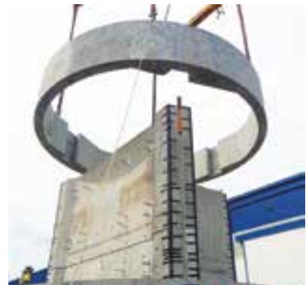
Precast & assembly of seawater intake tank for Chevron
