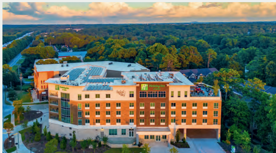
Holiday Inn & Suites Atlanta Perimeter – Dunwoody opened in 2021, complete with on-site photovoltaic solar panels to generate electricity and solar thermal panels for hot water, producing 15% of the hotel's energy use.
