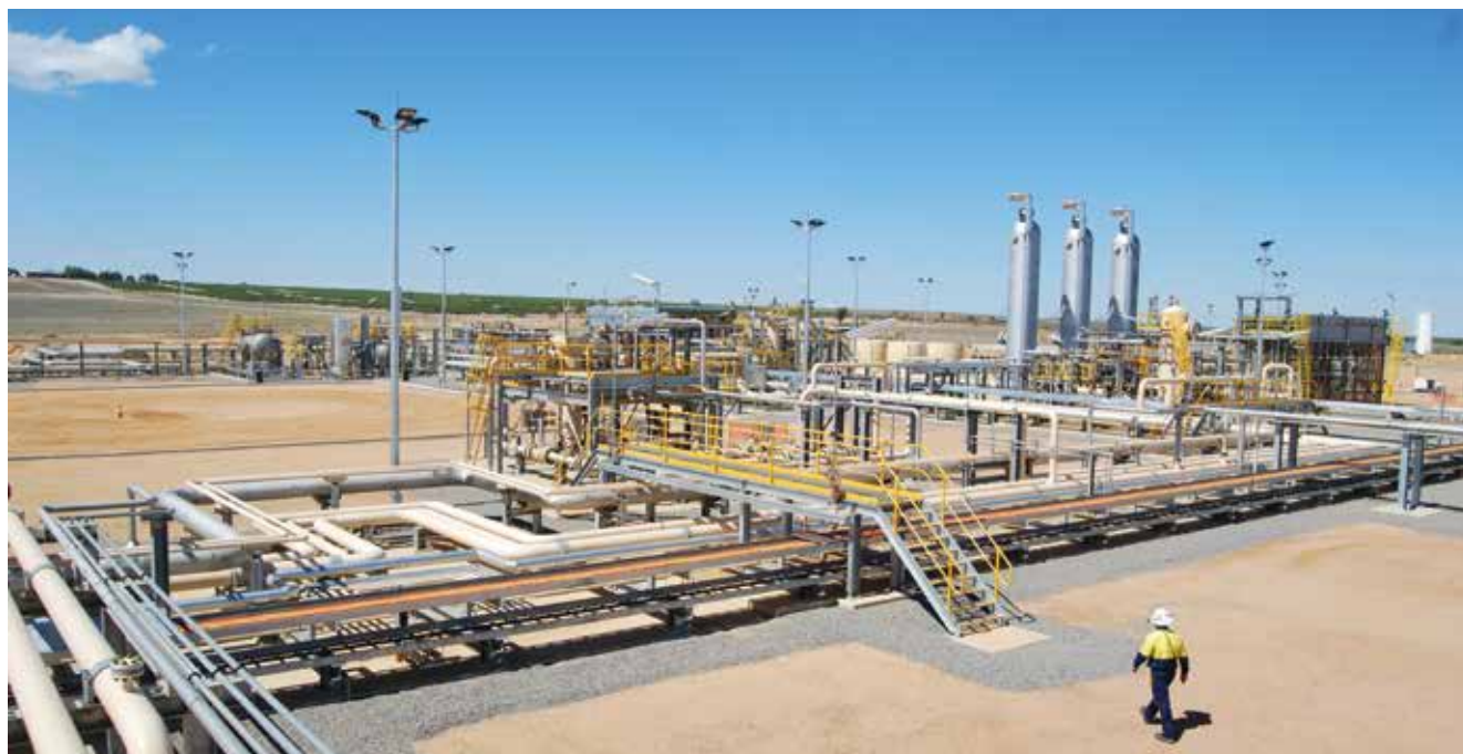
Storage capacity at APA's Mondarra Gas Storage Facility was increased during FY2016 with the completion of a new injection/withdrawal well.
